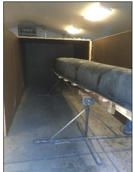
Figure 21: Curing Structure Under Construction
